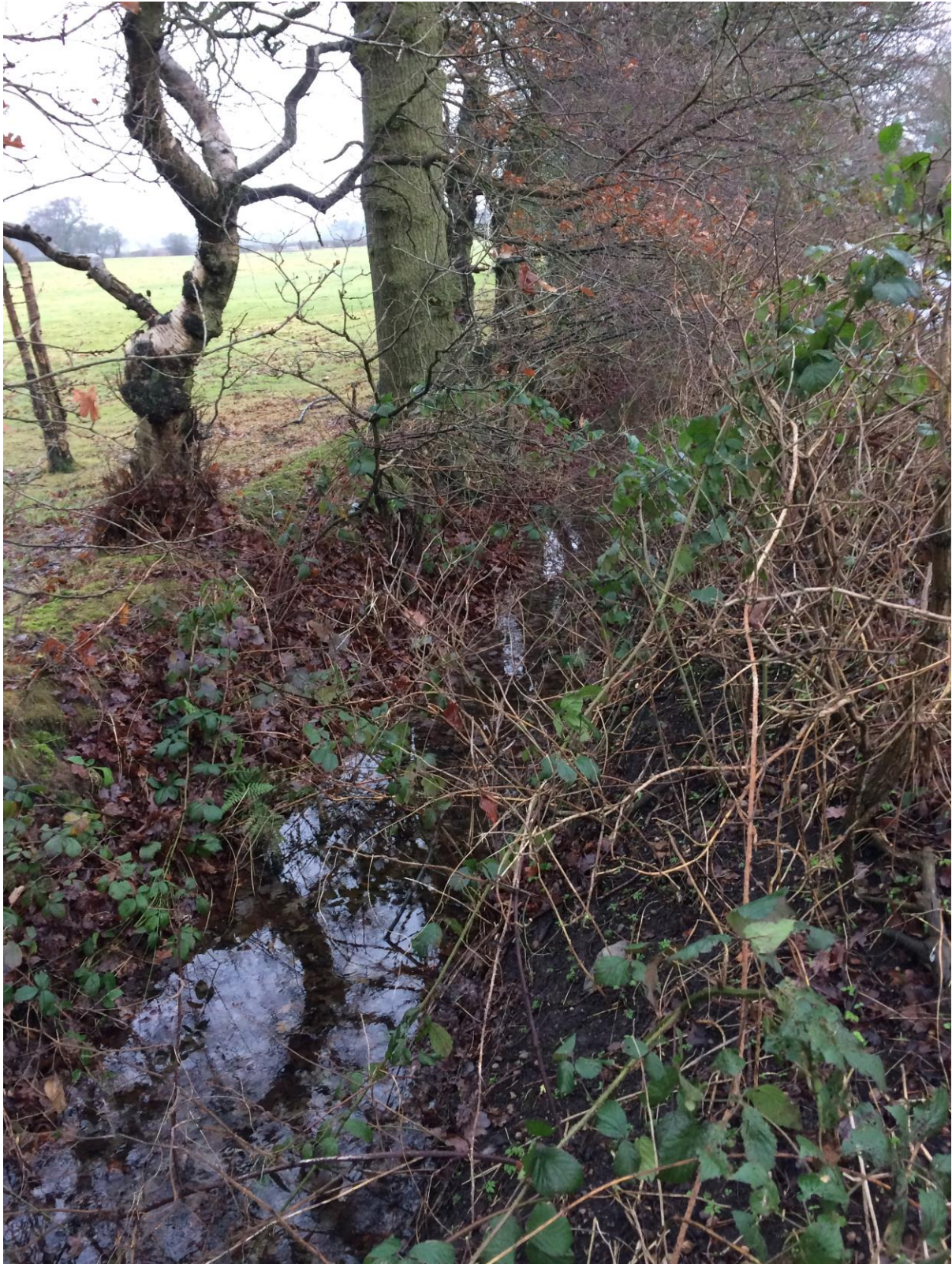
Outfall C (taken looking north from Straight Mile)
